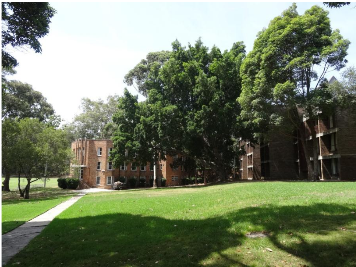
Figure 11: Reid (L) and Thyne (R) buildings looking south west
