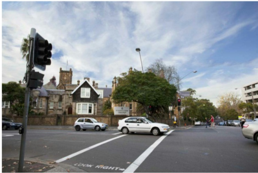
Figure 28: View of Vaucluse and Sulman Wings from Missenden Road and Carillion Avenue looking east
