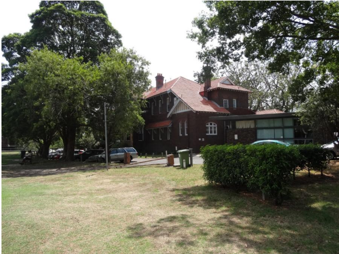
Figure 14: View of Harper building (L) and Angus Hall (R) looking north
