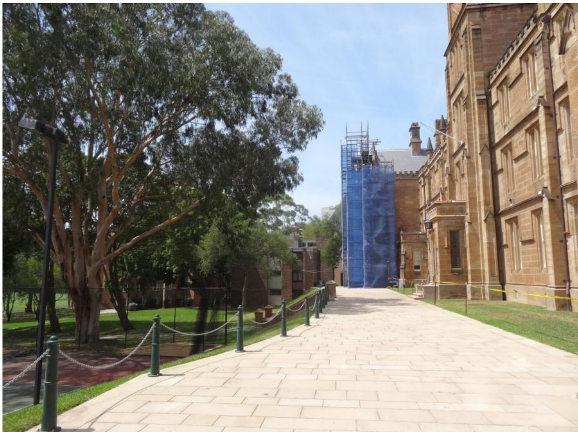
Figure 5: Looking south along the Main building forecourt
