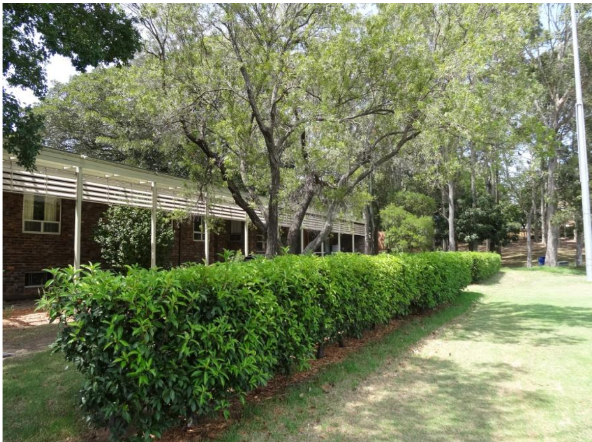
Figure 15: Existing Principals residence looking south east
